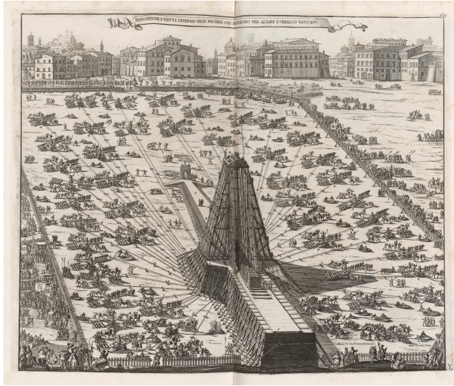
Figure 14: Carlo Fontana, Machinery used to lift the Vatican Obelisk in Rome in 1586, in Templum Vaticanum... (Rome: Giovanni Francesco Buagni, 1694), engraving, Montréal, McGill Rare Books.
