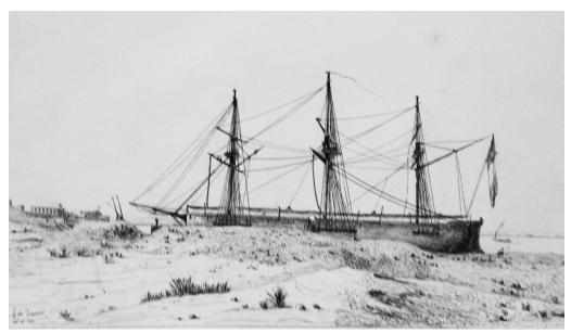
Figure 4: The Luxor, intentionally run aground, so the obelisk could be loaded into its hull
