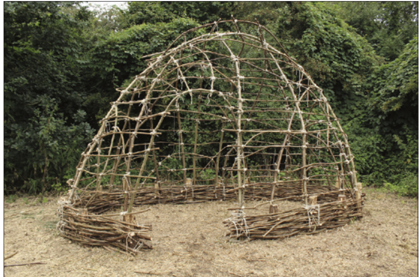
Fig. 6 Hut structure of the kind that may have been used at Nijmegen-Rust Wat: a spherical skeleton of branches on top of a vertical wicker substructure. – (After de Raaff 2018, fig. 3).
