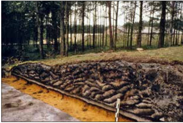
Fig. 3 This cross section of the barrow »Partisaensberg« near Kasterlee (prov. Antwerpen/B), in the Campine region, displays clear podzol profiles both below and at the surface of the barrow, which is built up of heath sods. – (Photo R. Langohr, Vakgroep Geologie en Bodemwetenschappen, Universiteit Gent).
