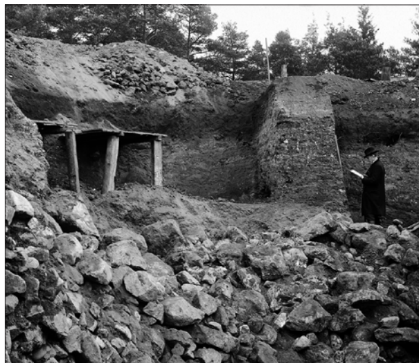
Fig. S2 Part of the crossing profile is documented (the major part had been excavated when the photo was taken). – (After Almgren 1905; ATA, RAÄ).
