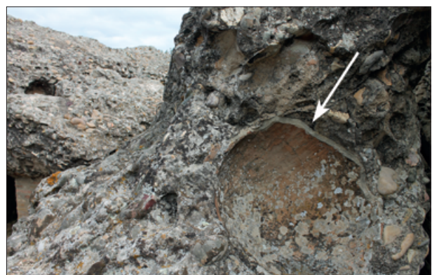
Fig. 8 Italica, Casa de la Exedra. Detail of oil amphora (Dressel 20) embedded in the opus caementicium of the exedra . – (Photo R. Hidalgo-Prieto).
