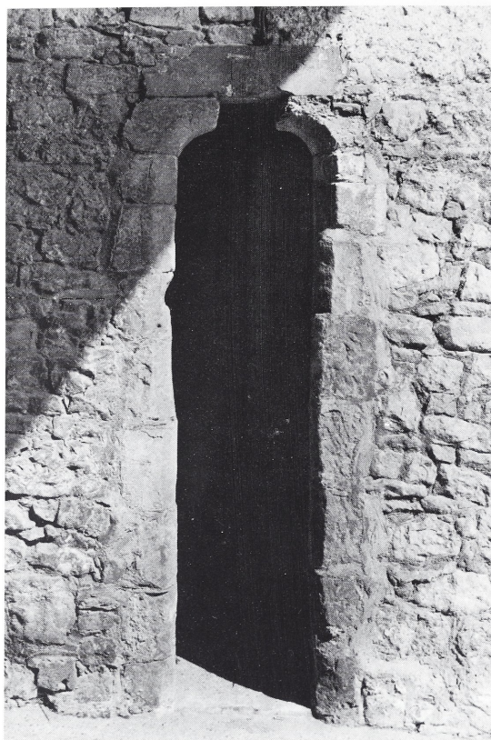
Fig. 18 Nettlestead Place, Nettlestead, Kent, England. Door with shoulered arch giving access to lower chamber of Gate House, 14th century (Photo: Country Life).
