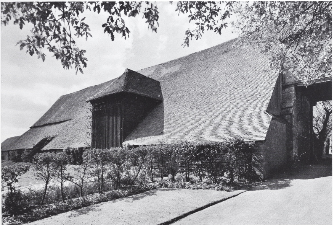
Fig. 15 Nettlestead Place, Nettlestead, Kent, England. Manor Barn with Gate House, Exterior from east (Photo: Country Life).
