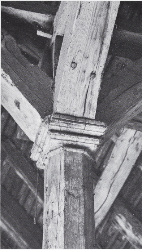
Fig. 17 Nettlestead Place, Nettlestead, Kent, England. Gate House, 14th century, detail of king post in room over gateway (Photo: J. W. Roberts).
