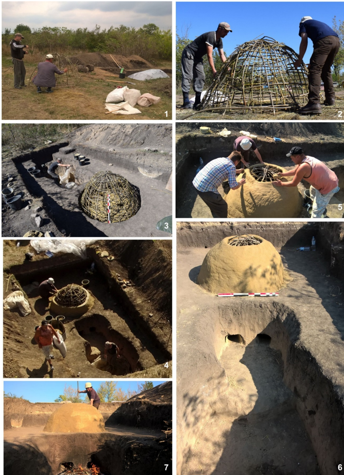
Pl. III. Construction of the experimental kiln: 1-3. Building the wicker frame of the vault; 4-5. Raising the vault in the technique of wattle and daub, with clay mixed with chaff and water; 6. The kiln; 7. Drying the kiln (photos by the authors).
