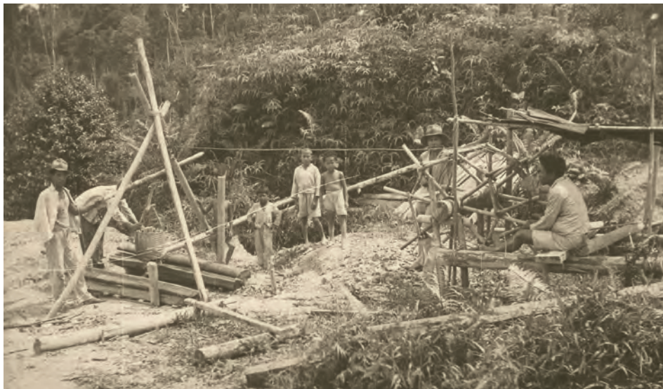
Fig. 1 Baskets full of ore are pulled from a shaft using a self-made wooden reel with a rope winch, Tewah/Kalimantan, photo by Karl Helbig, 1937 (Roemer- und Pelizaeus-Museum Hildesheim).
