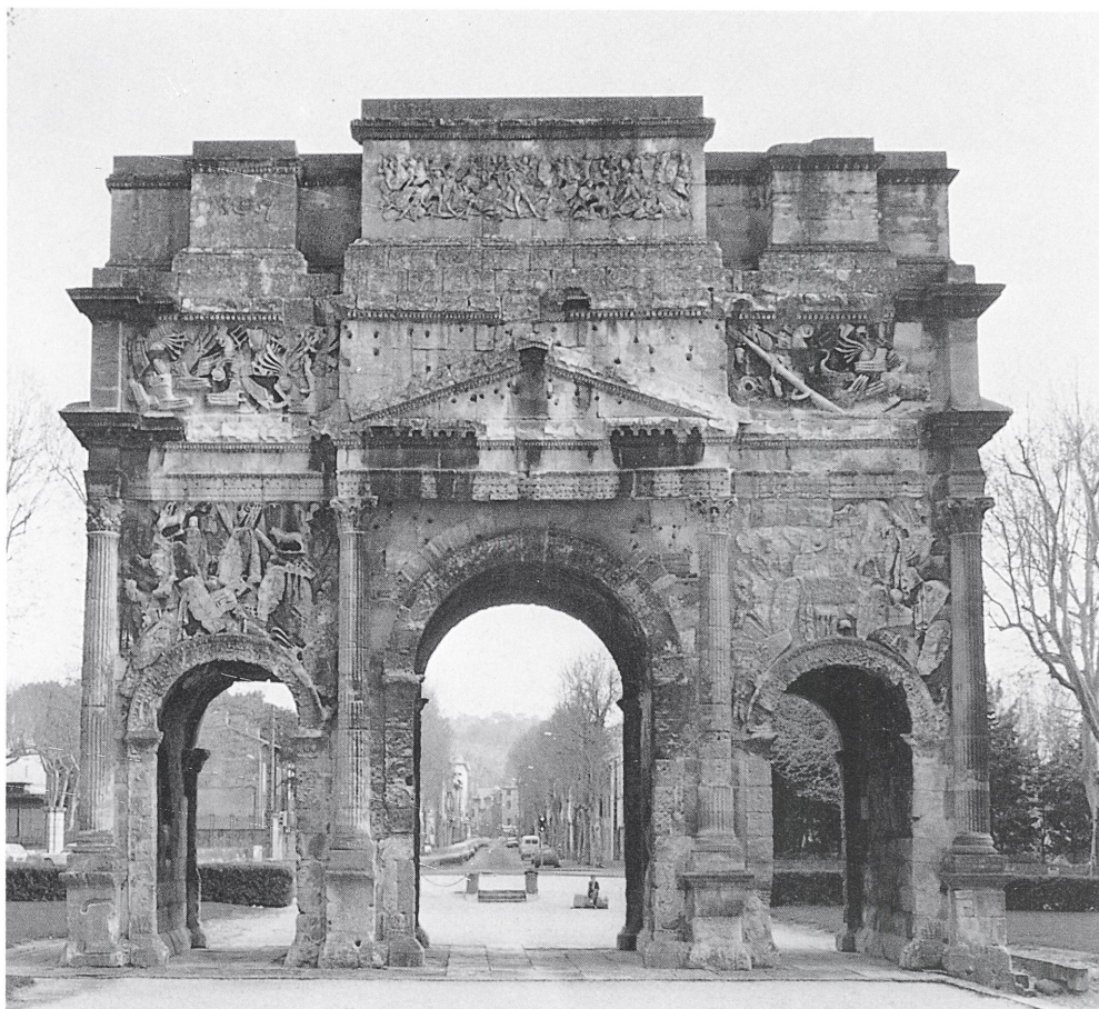
1 Arch at Orange, north face.
