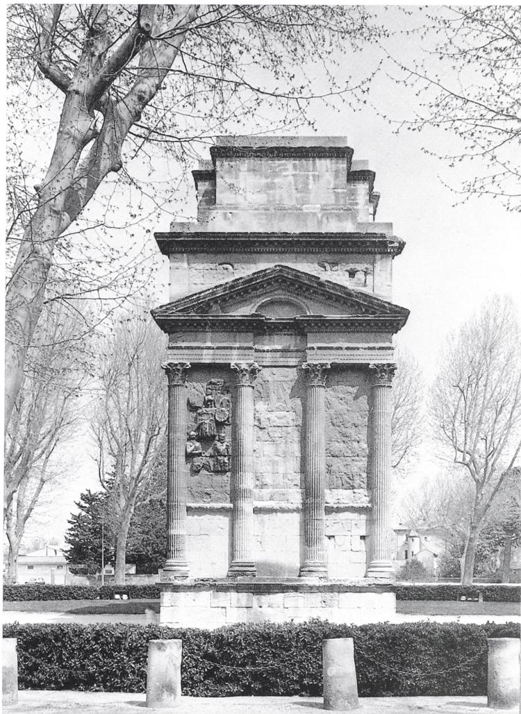
11 Arch at Orange, narrow west face.
