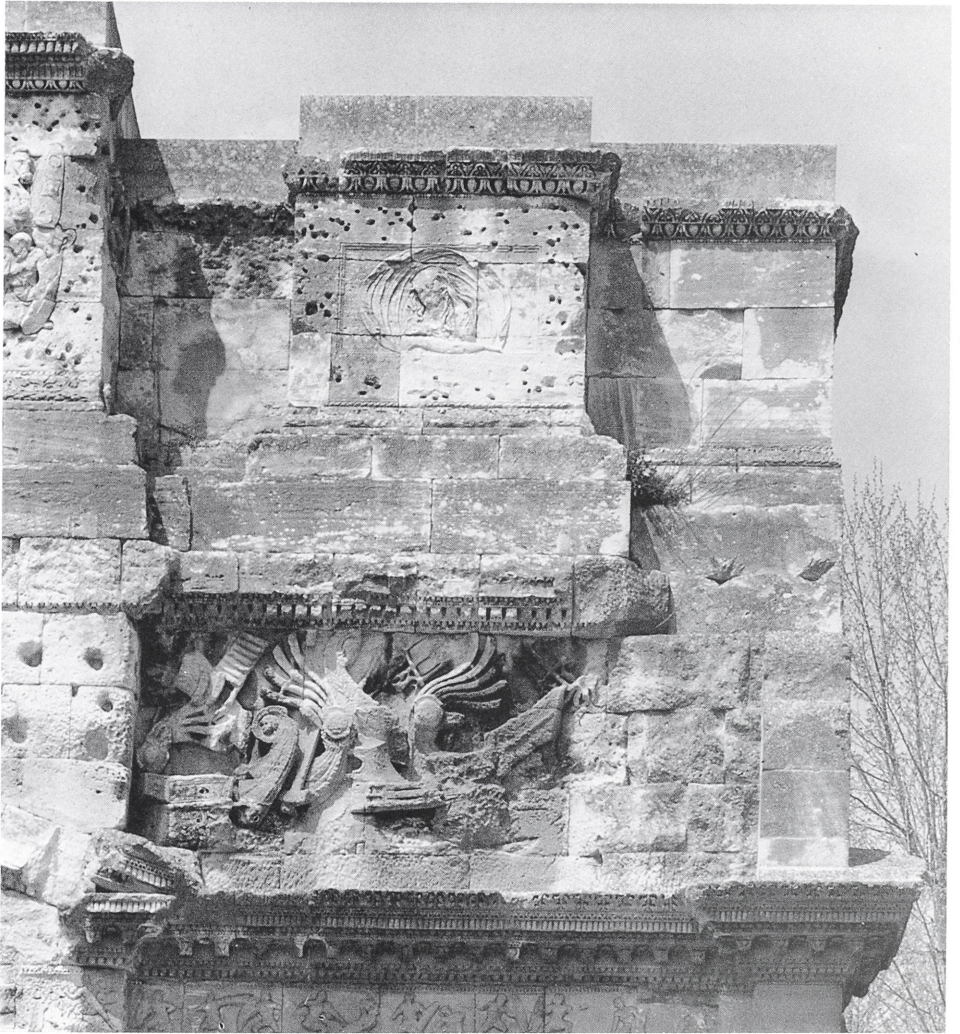
17 Arch at Orange, southeast face, detail.
