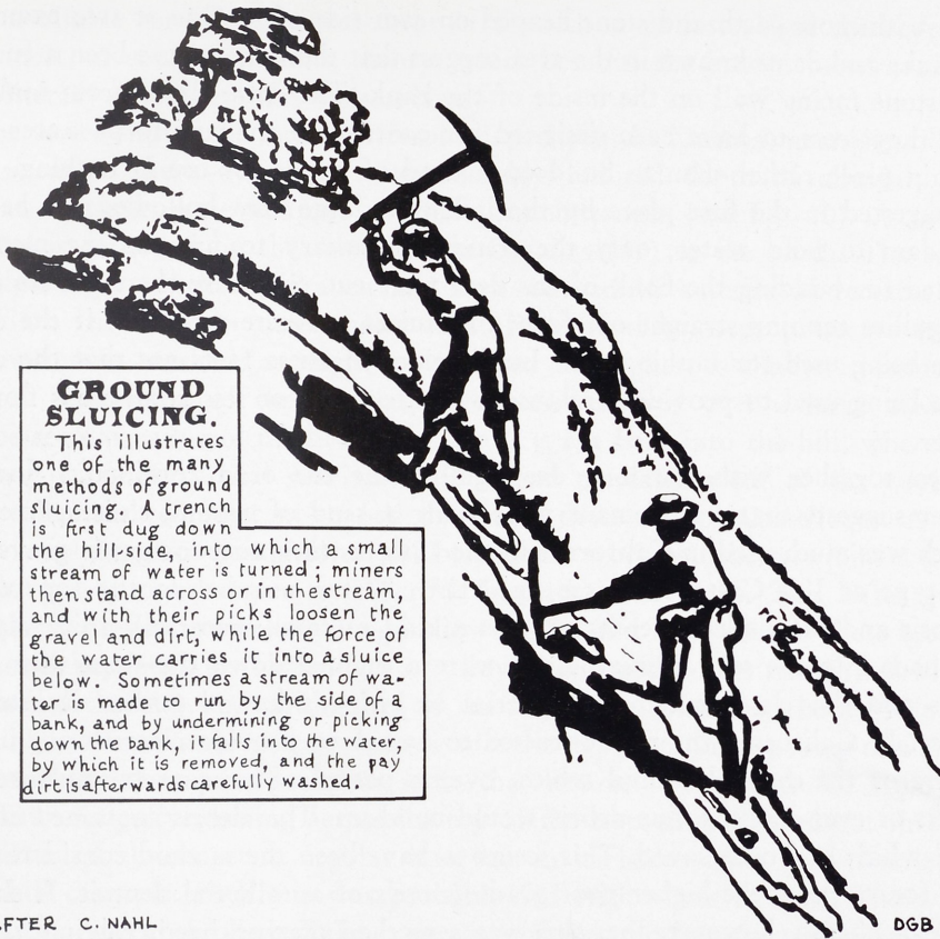
11 Ground sluicing in nineteenth century California.
