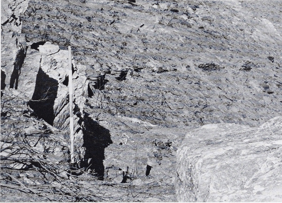
17 Cabrera valley: rock cut and built up aqueduct supplying the mine at Las Médulas. (Photograph by the author.)
