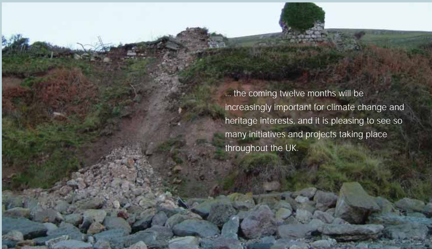
Collapse of medieval masonry from coastal erosion at Gogarth Grange, Great Orme, Llandudno. Credit: Gwynedd Archaeological Trust
