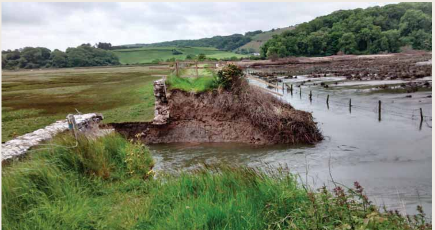
Photograph showing the breach in the bank and where the phases of construction can be seen. Credit: Judith Doyle
