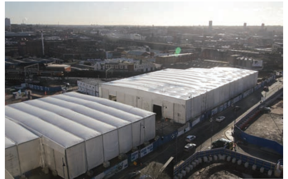
Bird’s-eye view of excavation tents looking south west. Credit: LMJV
