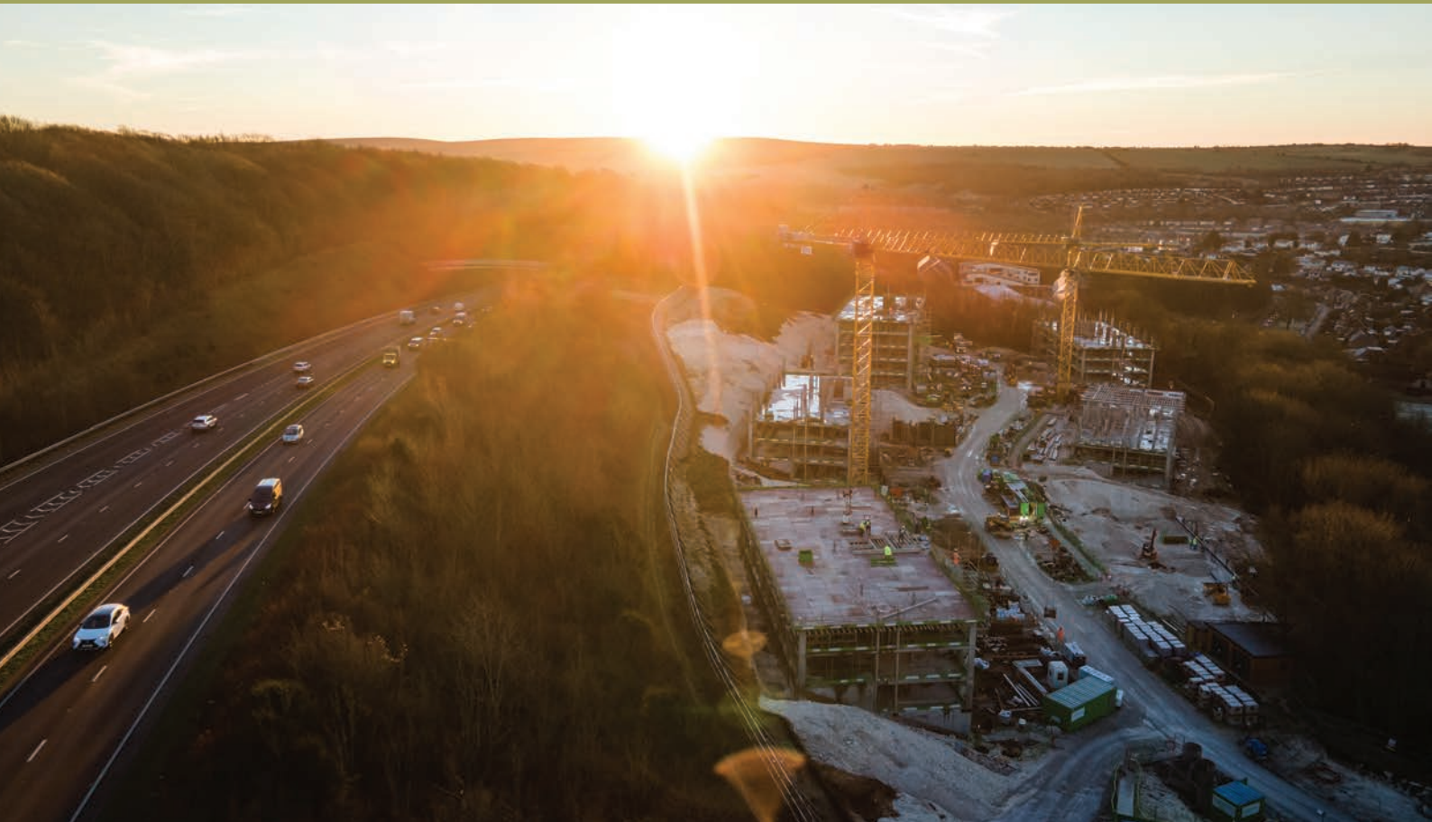
Aerial view of busy construction site in morning sunlight close to Brighton, East Sussex, UK. Credit: P Babic (Shutterstock)
