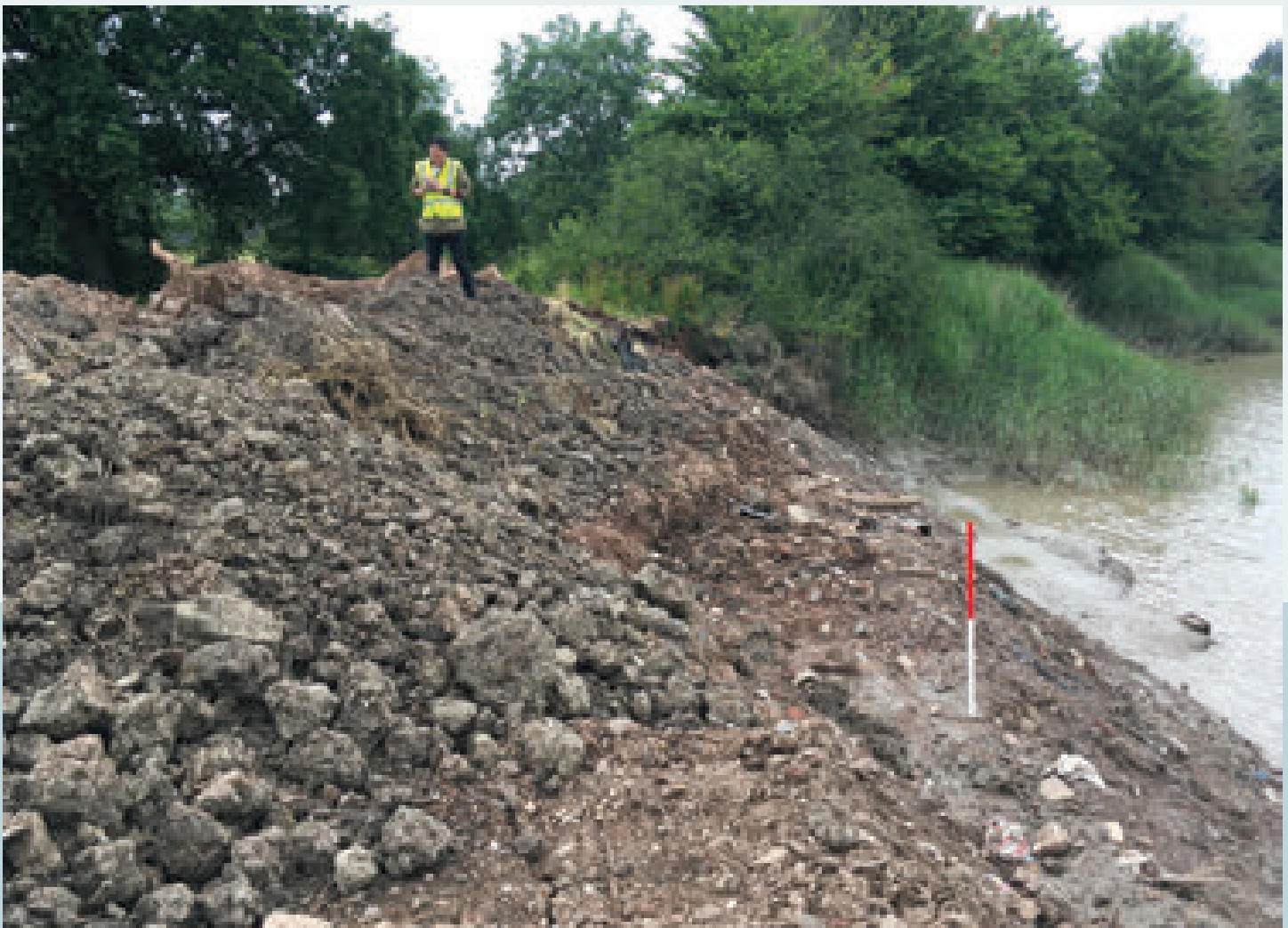
Cadw site inspection of tipped material adjacent to Caerleon Roman legionary fortress and amphitheatre. Credit: Cadw
