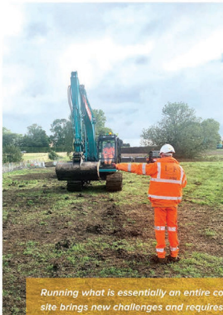
L – P: Archaeology staff working as bankers to safely oversee the movement of plant and delivery lorries. Credit: L – P Archaeology; © HS2 Ltd
