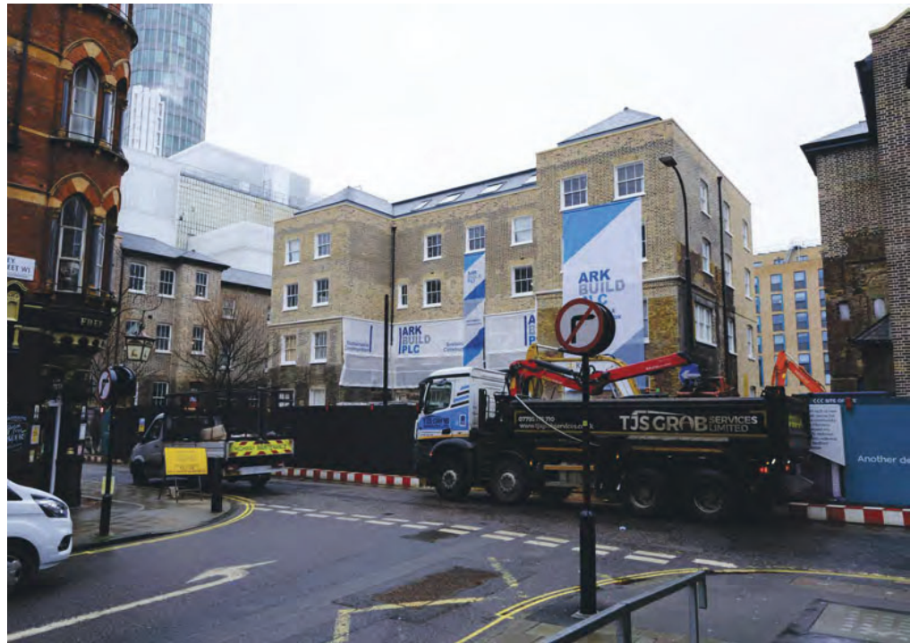
Retained workhouse. Credit: Icen Projects
