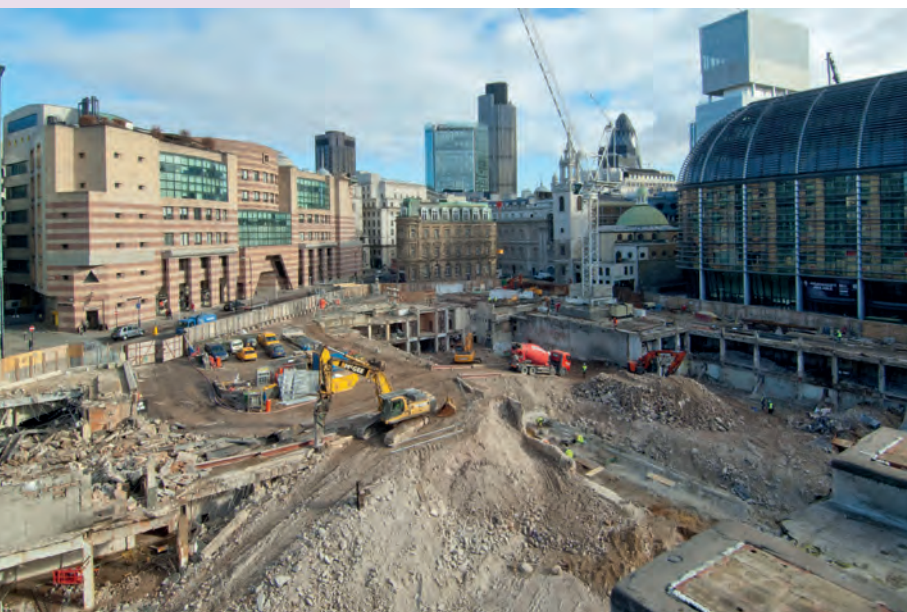
Bloomberg construction site during demolition (Photo: MOLA)
