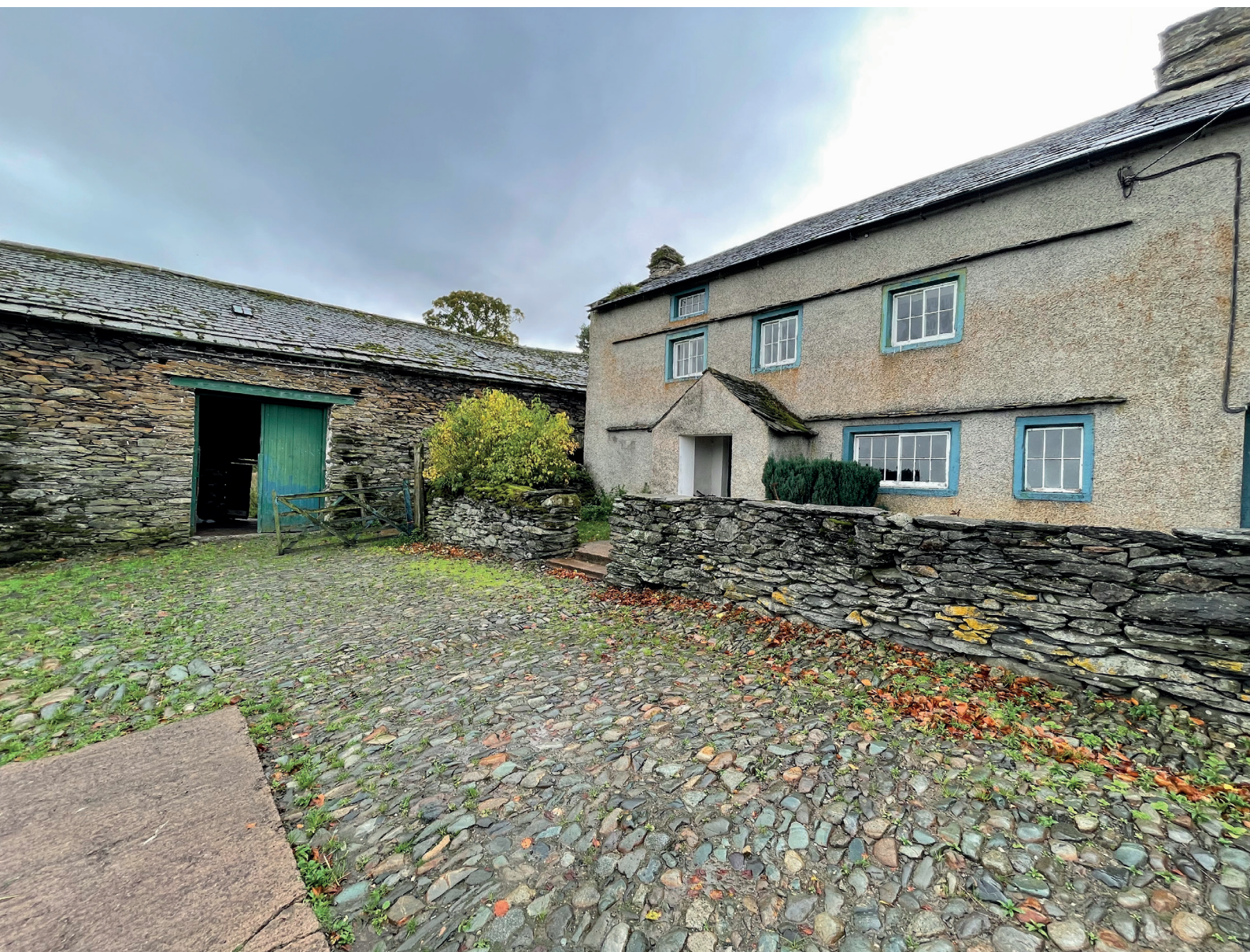
Front elevation of the farmhouse, with the south barn to the left ©www.parti.global
