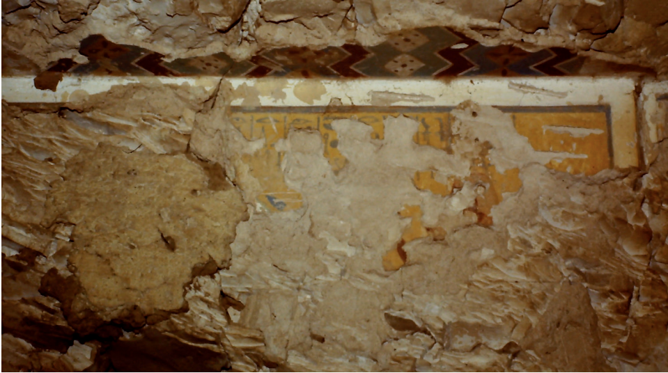
FIG. 6: View of the right lintel in TT 118.
