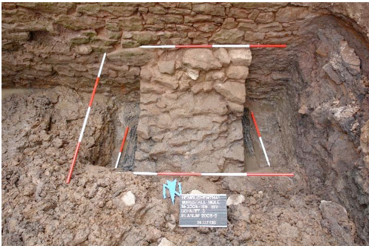
Picture 14: One of the two stabilizing pillars built in front of the circular wall.
