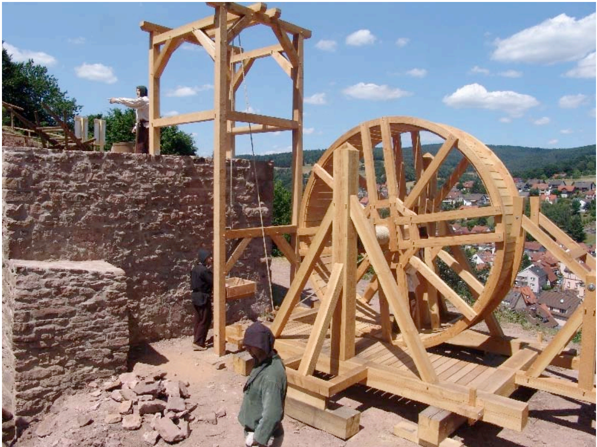
Picture 04: A medieval construction site with a treadwheel could be visited during the festivities on the castle “Bartenstein” near Partenstein in 2009.
