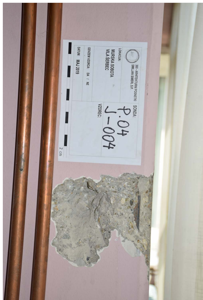
9 Research of the structure on the pier: determining the preservation of the primary piloti under the secondary layer of concrete. Photo: Smiljan Simerl, 2019
