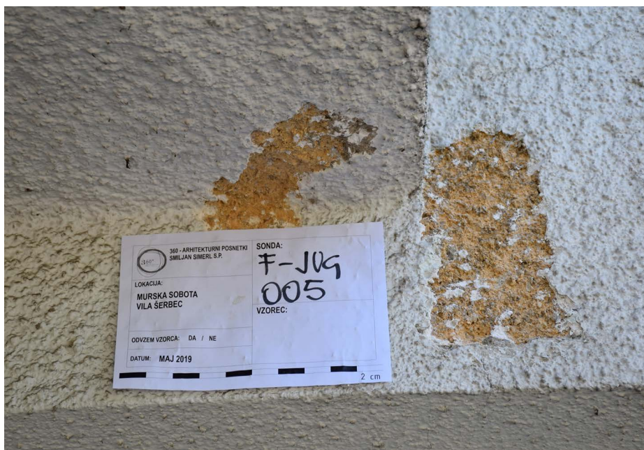
8 Research of the structure – façade: identification of the colour tone and plaster texture. Photo: Smiljan Simerl, 2019
