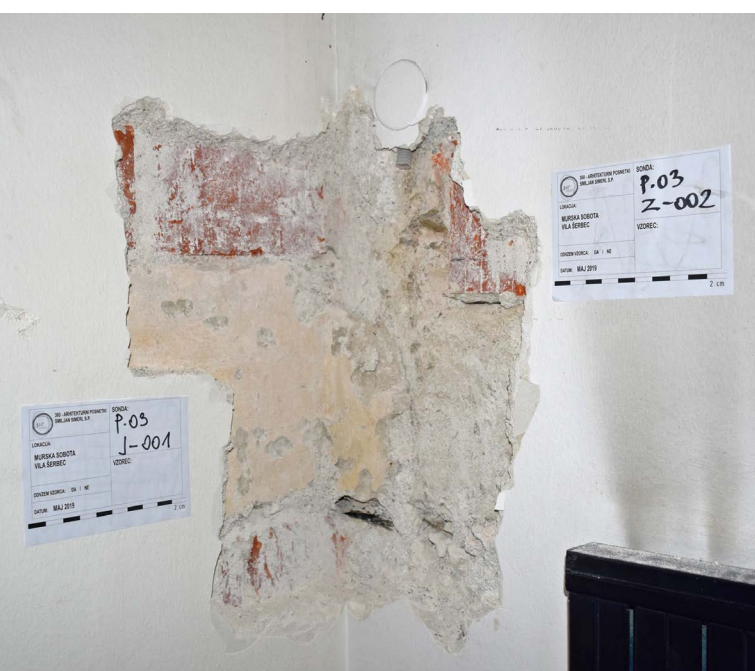
10 Research of the structure in the area of the staircase: checking the possibility of the existence of a single-armed staircase. Photo: Smiljan Simerl, 2019
