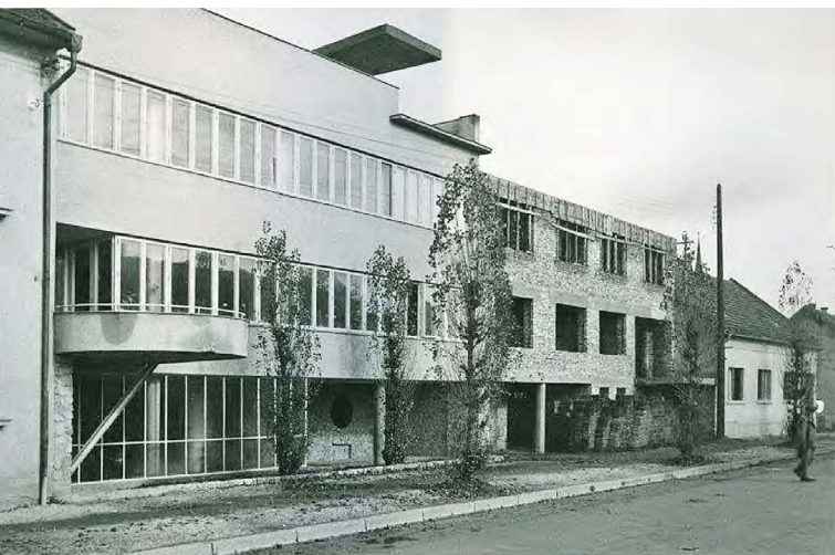
3 Façade of Villa Šerbec. Undated photograph
