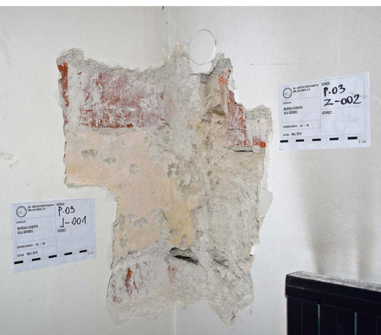
10 Research of the structure in the area of the staircase: checking the possibility of the existence of a single-armed staircase. Photo: Smiljan Simerl, 2019
