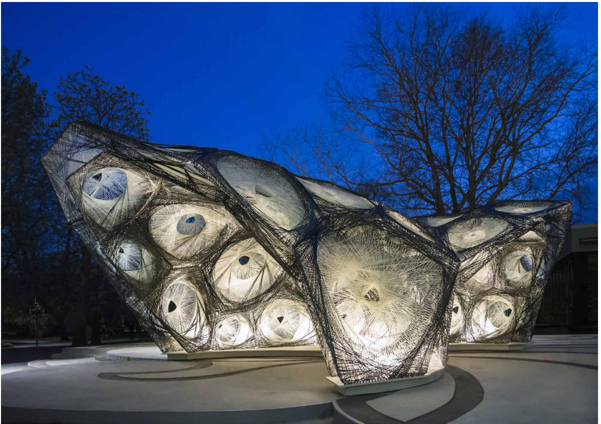
Figure 3: ICD/TKE Research Pavilion 2013-2014 , Institute for Computational Design (ICD, Prof. Achim Menges) and Institute of Building Structures and Structural Design (ITKE, Prof. Dr.-Ing. Jan Knippers) at the University Stuttgart. Based on the differentiated trabeculae morphology and the individual fiber arrangements, a double-layered modular system was generated for implementation in an architectural prototype. ©ICD/ITKE Universität Stuttgart.
