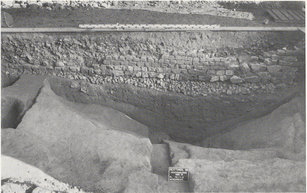
Fig. 3 Wall 37 of Bau M with several phases overlying the filling of the outer ditch of Kastell V. To reduce possible sinking of the wall, a slightly stronger foundation was built here. The ditch was cut into the natural clay.
