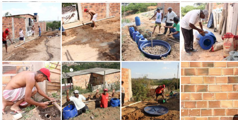
Figure 5 - Construction of the Evapotranspiration Tanks
