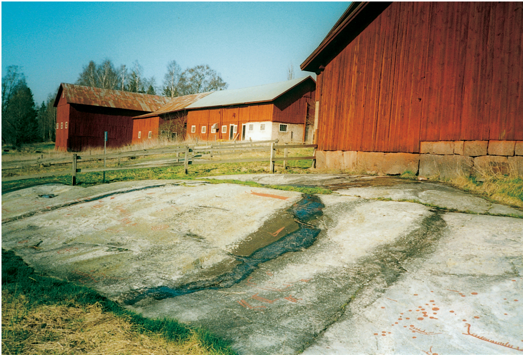
Fig. 5. Site A with staining of the surface, barn immediately above the carved surface.
