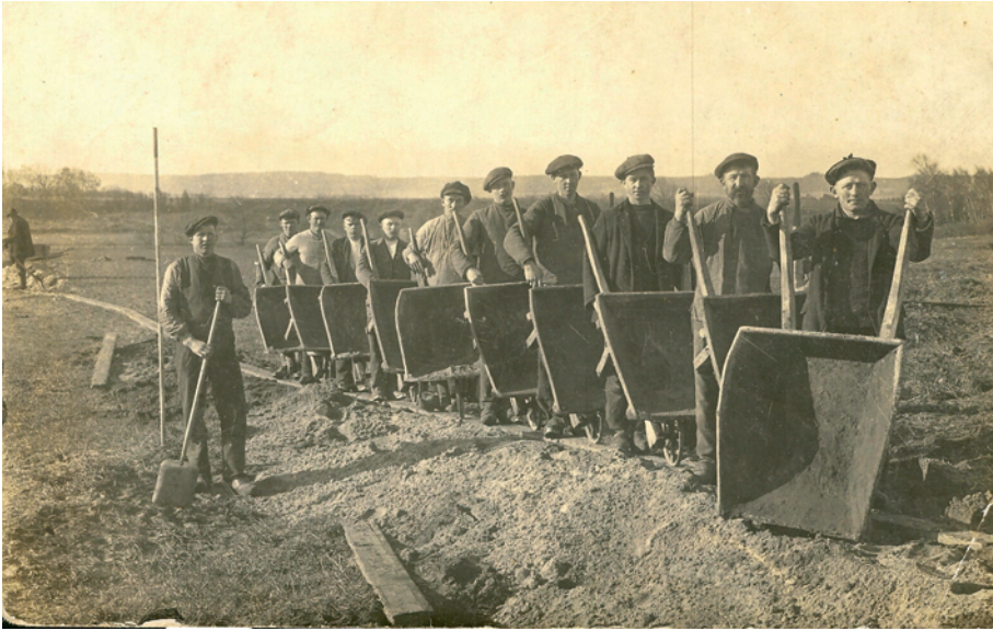
Fig. 6. Workers with their shovels and wheelbarrows during the construction of the hydro-electric power plant at Tange.
