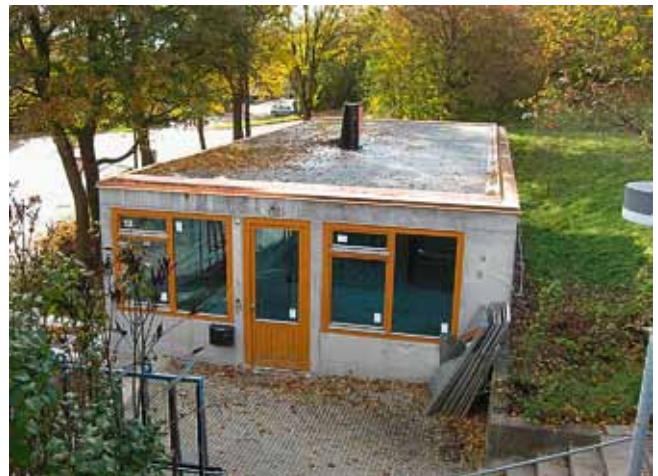
Gatekeeper's house with copper edging to the roof and highly reflective blue windows on the façades 2010 (photo: Monika Maus)
