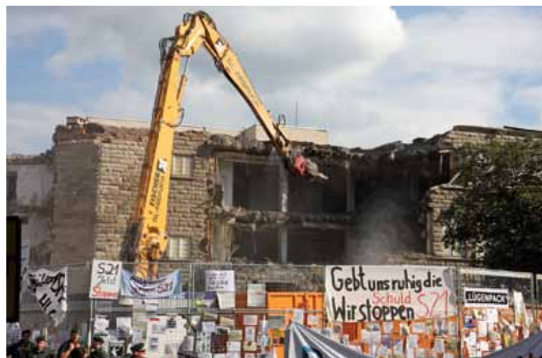
Stuttgart Central Station, demolition of the north wing (photo: R. Vogler)
