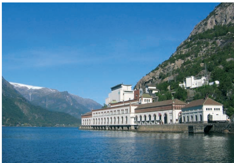
The Tyssø hydropower plant (1906-16) is today a national monument and beautifully restored after its closure in 1996 (Photo: Axel Mykleby)
