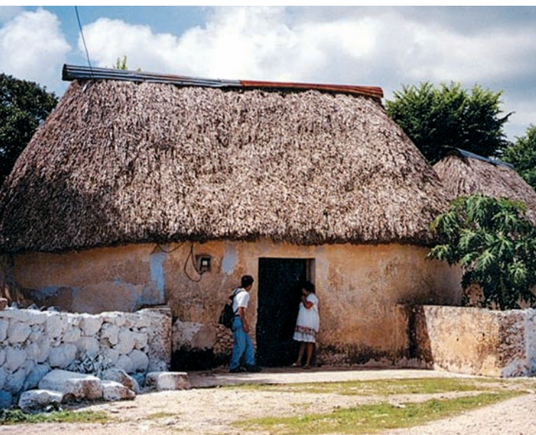
Adobe house with thatched roof
