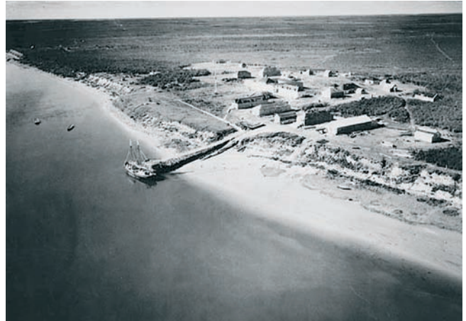
Historic image of York Factory with its complex of associated buildings and structures, circa 1925 (Library and Archives Canada, PA-041571)
