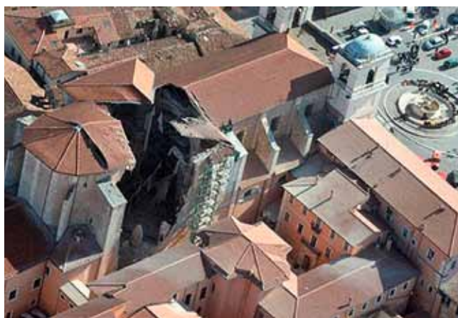
L'Aquila, aerial view of the damaged cathedral
