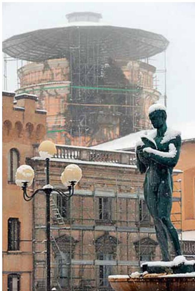
L'Aquila, Santa Maria del Suffragio, dome with temporary roof
