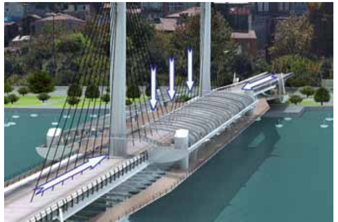
Figs. 7 and 8. The project of the Halice Metro Bridge (1999) has grown since 2002. It is now presented as a multifunctional cable-stayed bridge, almost 20 m above the sea with two pylons almost 70 m high. The bridge will be 390 m long with a 180 m long Metro station on top.
