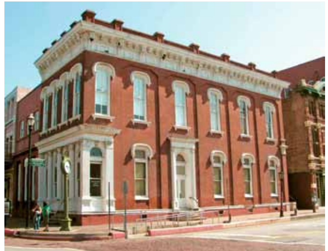
Galveston, Texas, typical late 19th century building
