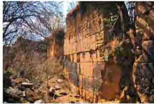
Inner wall of Chubjakha Dzong, Paro
