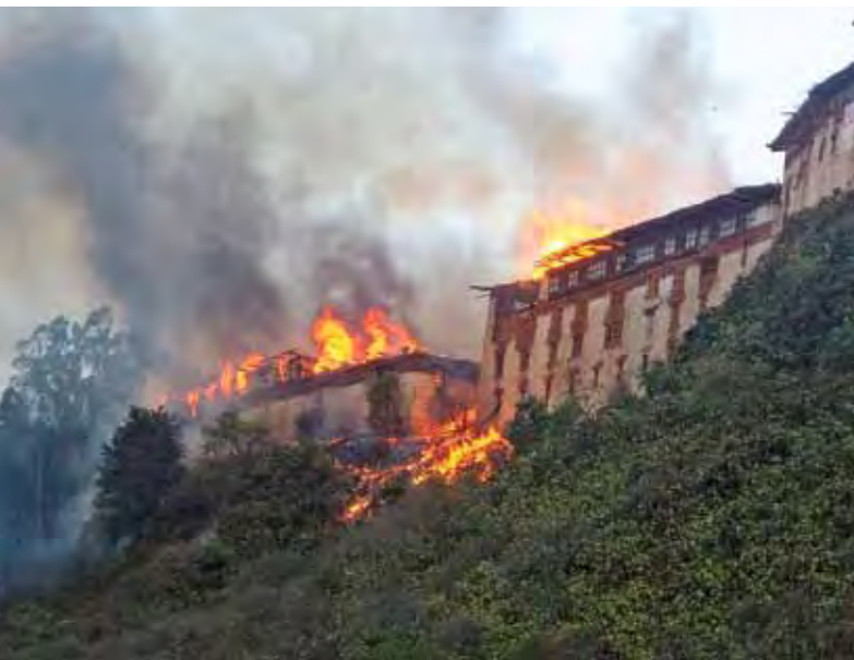
Wangduephodrang Dzong, the fire of June 24, 2012 (photo: Dawa Knight)
