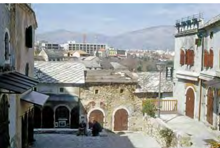
reduce the unacceptable visual impact of the new structure of the Hotel Ruza;
