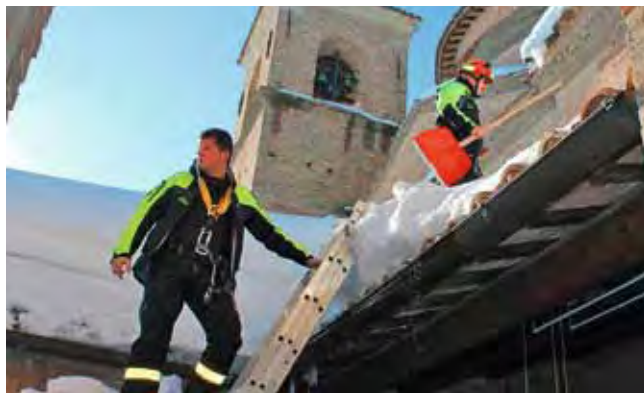
Urbino, Marche, removing snow from the roof of San Bernardino monastery
