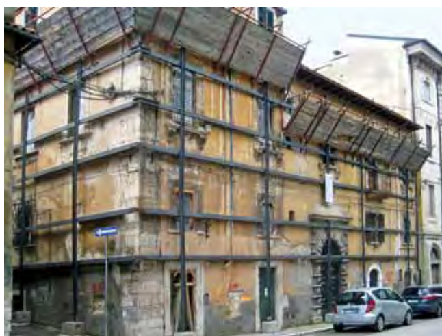
Ongoing repair work in L'Aquila (photos: www.dorsetdaze.wordpress.com )
