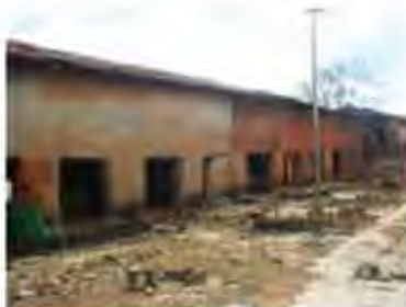
Photo 12. Internal corridor of the palace
