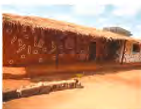
Photo 7. The outside of the Obatala shrine after restoration.
