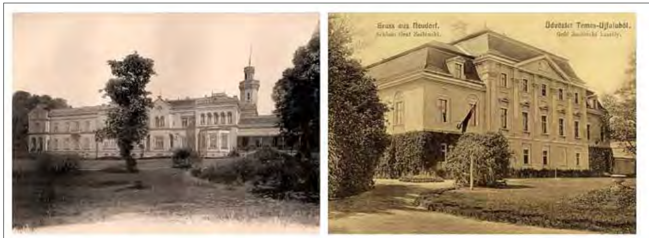
The Csité-Csekonics Manor House (Jimbolia, Timiș County; left) from the late 19th century and the Zselensky Manor House (Neudorf, Arad County; right) from the early 20th century
