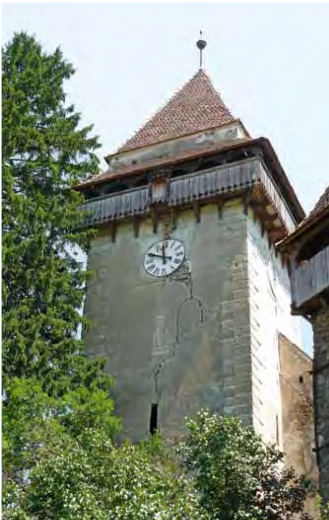
Apold/Trappold, fortress before and after the restoration
