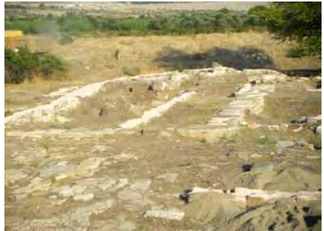
Allianoi, sandfill completed
