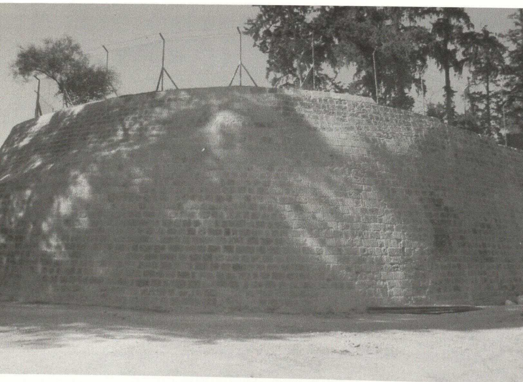
The Roccas bastion after conservation
