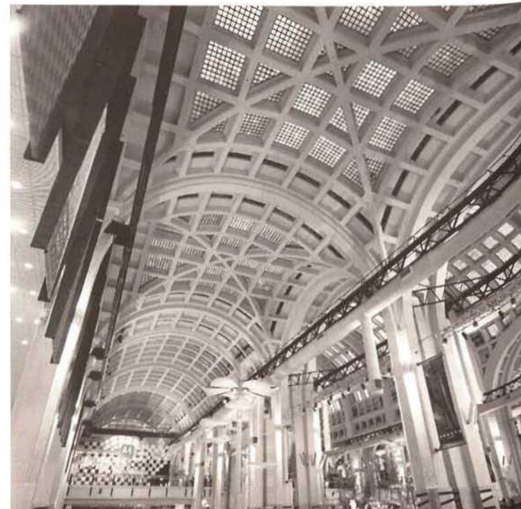
Abasto Market, Buenos Aires, 1929–32. Interior after renovation
