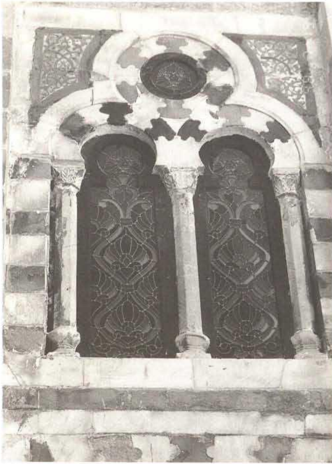
Azhar Mosque in Cairo, Fatimid Riwaq after “restoration”: new reinforced concrete base with marble facing (complete renovation)
