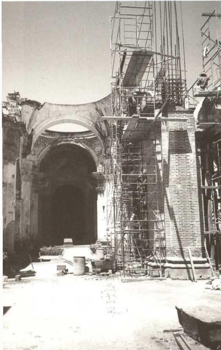
Antigua Guatemala, partial reconstruction of the cathedral, damaged by an earthquake
