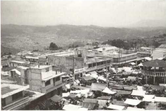
San Francisco El Alto, market place. Almost all the traditional houses have been replaced by new reinforced concrete buildings.
