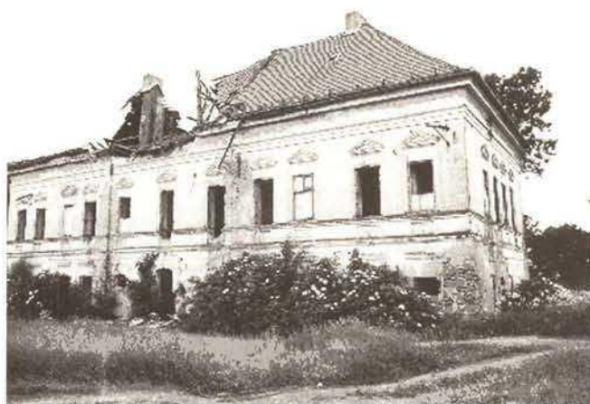
Žip, neo-classical manor house with collapsed roof
