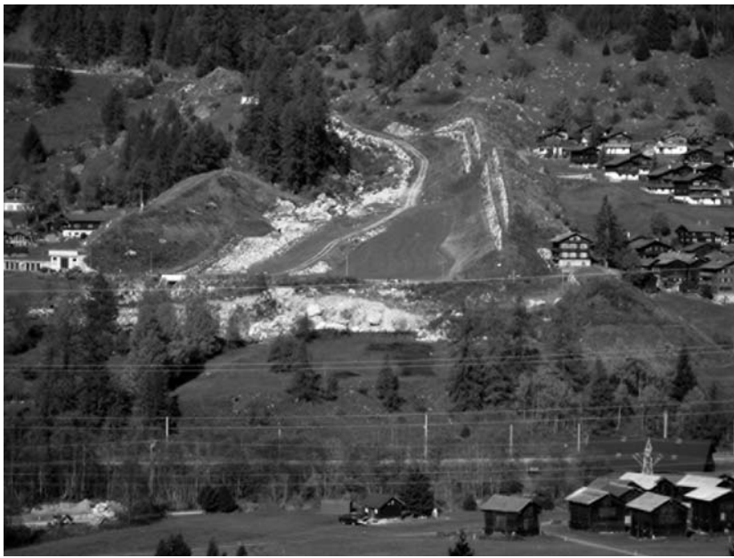
Fig. 2 Avalanche protection dams near Selkingen, canton of Valais
