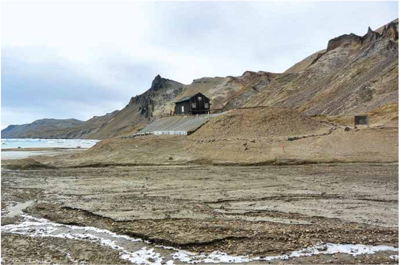
Fig. 3: Snow Hill historic hut in Antarctica showing an attempt to stop increasing erosion of the gravel mound it sits on (photo Mike Pearson)
