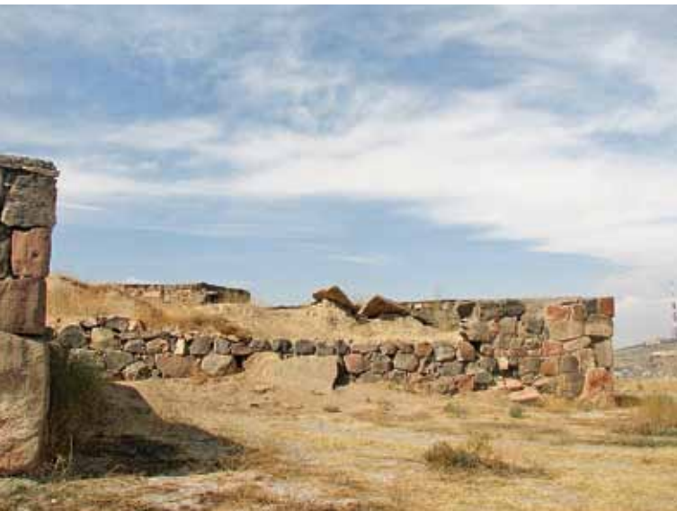
Ruinous state of the surrounding walls
